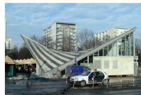
Warszawa Ochota train station in Poland (Source: [Z06])
