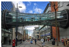
Corporation Street Bridge. (Source: [Z05])
