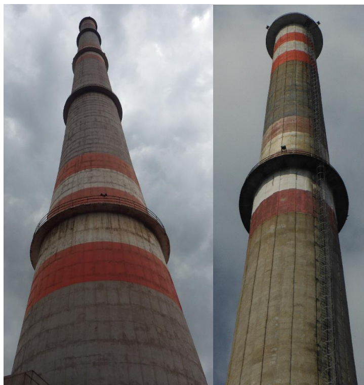
Figure 3 - general view of the reinforced concrete shaft of the chimney constructed using folded formwork (left) and hydraulically extendable (right) formwork. [2]
