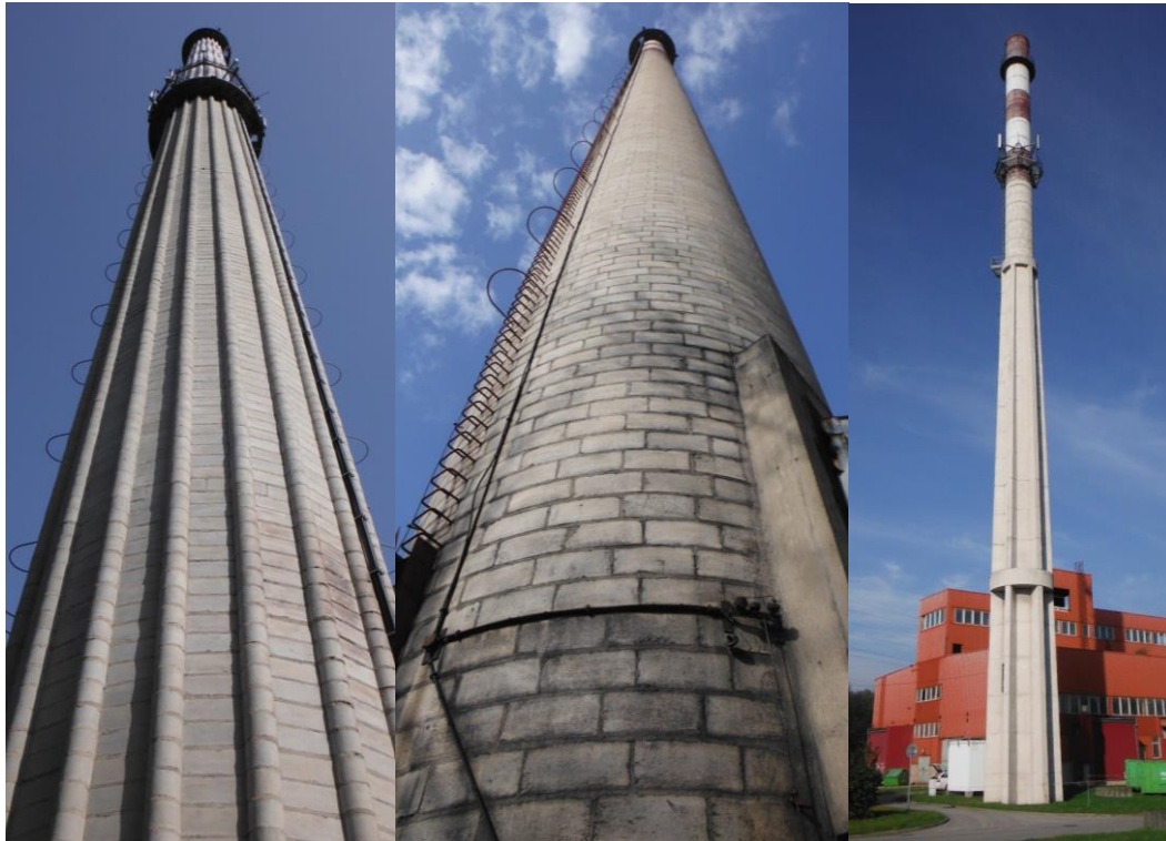
Figure 2 - general view of the chimney shaft type Monoyer (left), type "Z" (center) and type "T" (right). [2]
