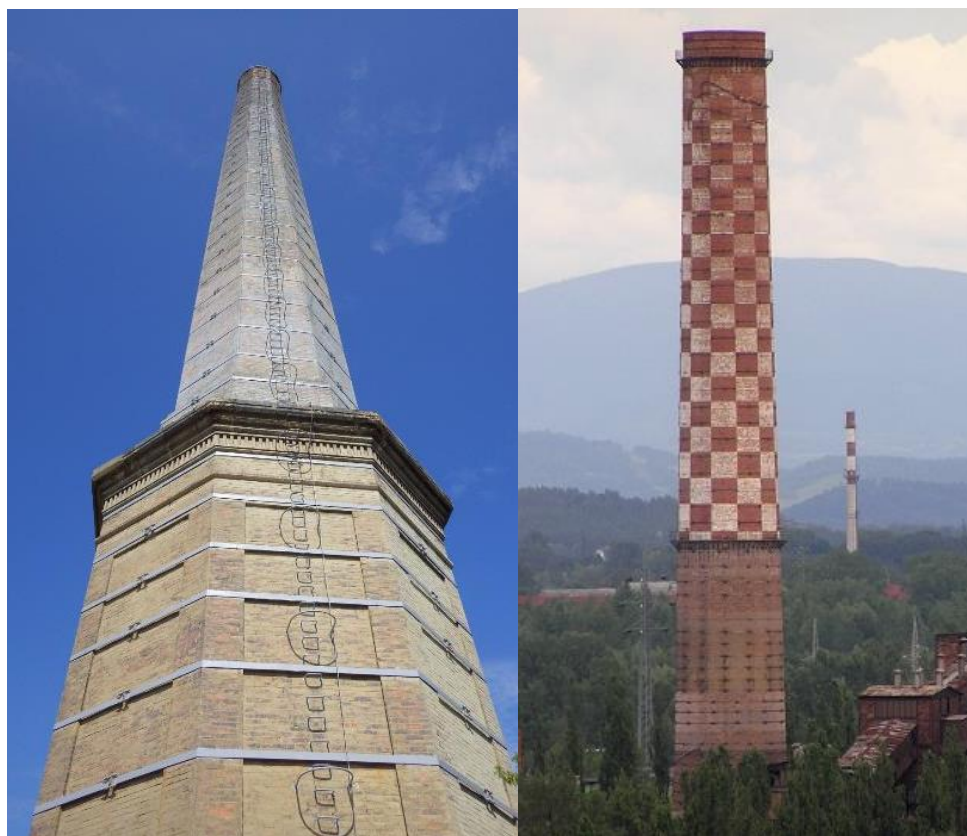
Figure 1 - general view of the brick shank of the chimney with octagonal cross section (left) and circular cross section (right) [2]
